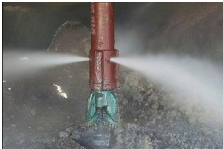
Figure 5-2.—Water separator discharging water before it reaches the drill bit.
